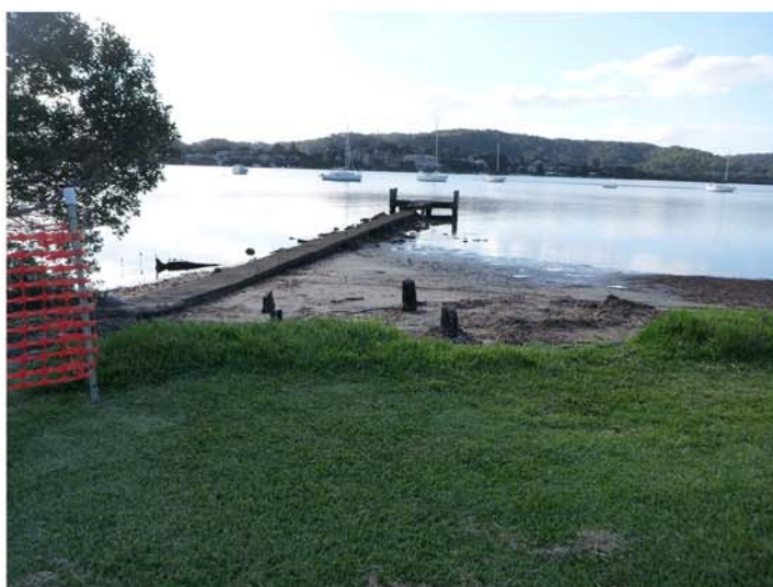
CONCRETE AND TIMBER JETTY
