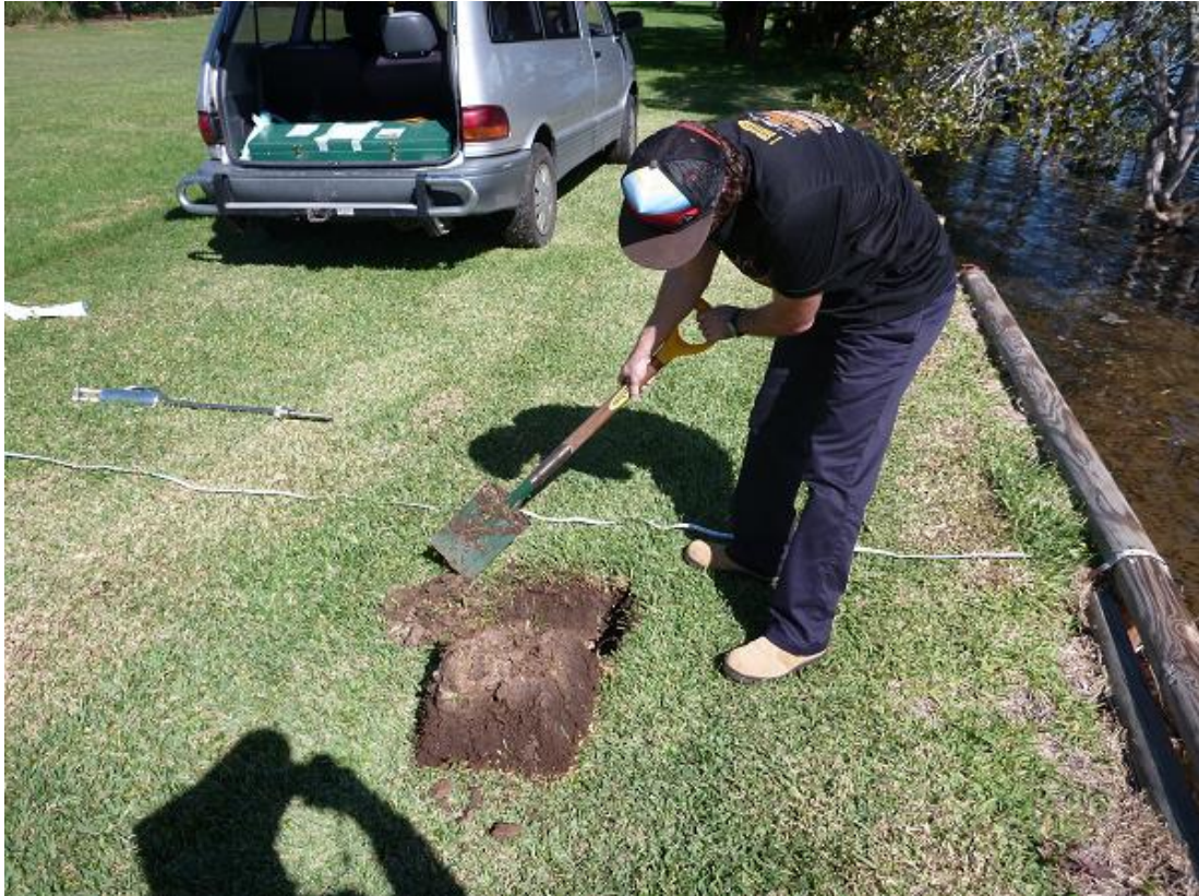
Photograph 1 – Test Pit behind the existing timber wall near the dilapidated jetty
