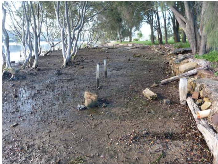
MANGROVES AND DETERIORATED ROCK AND TIMBER WALL
