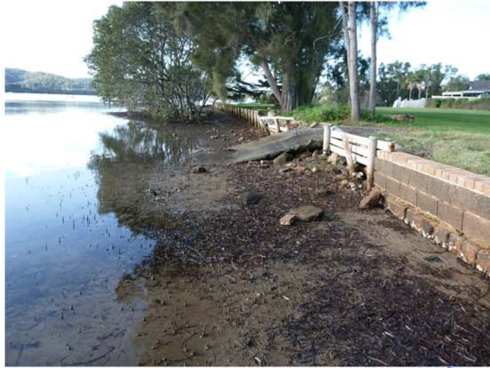
BLOCKWALL AND RAMP
