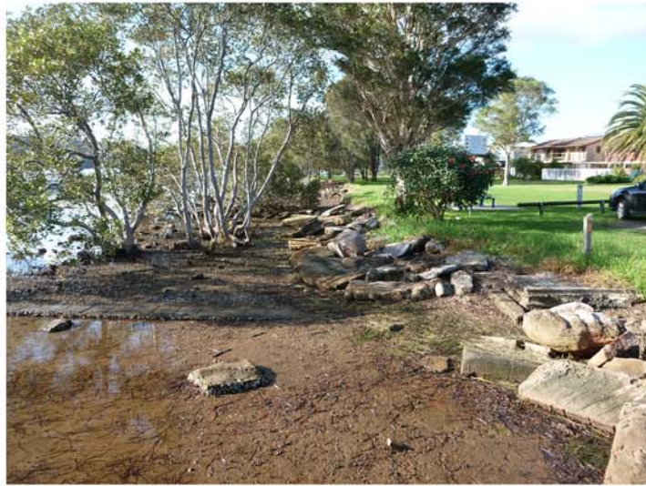
MANGROVES AND PLACED ROCK
