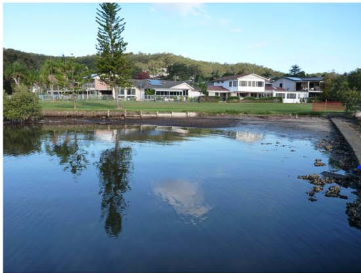
BEACH AND DETERIORATED TIMBER WALL
