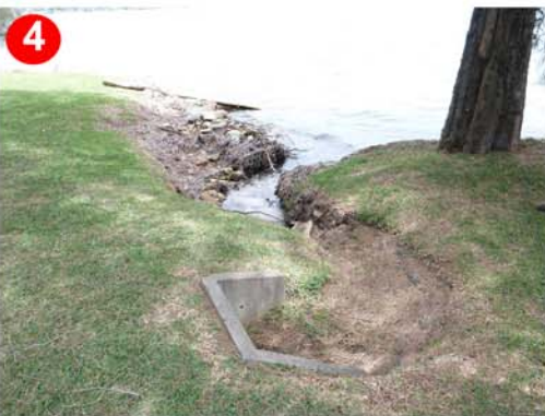
4 Pipe terminated behind seawall and dilapidated gabion
