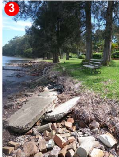
3 Brick and concrete rubble along foreshore
