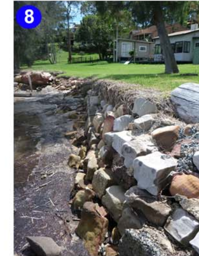
Mortared sandstone blockwork wall
