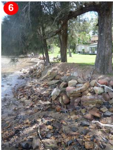
6 Casurinas exposed at base behind sandstone and concrete wall
