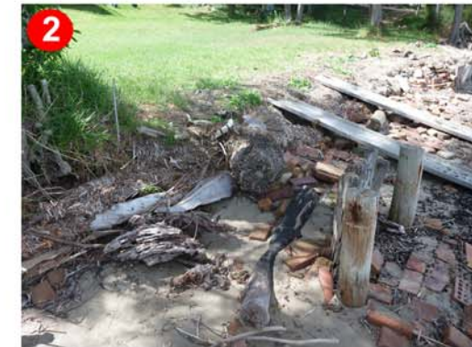
2 Aluminium ramps, vertical logs wall and brick and concrete rubble
