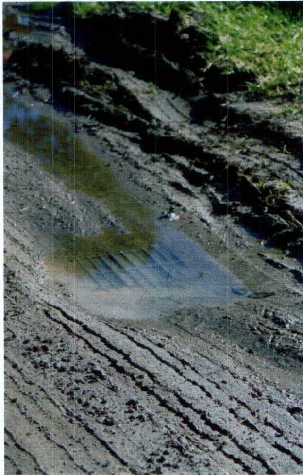
Figure 15: Blocked drains with sediment
