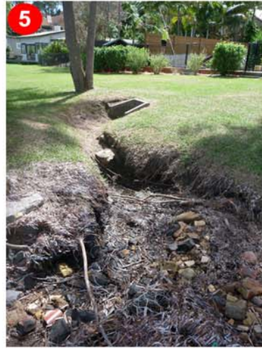
5 Pipe terminated behind seawall and dilapidated gabion in foreground
