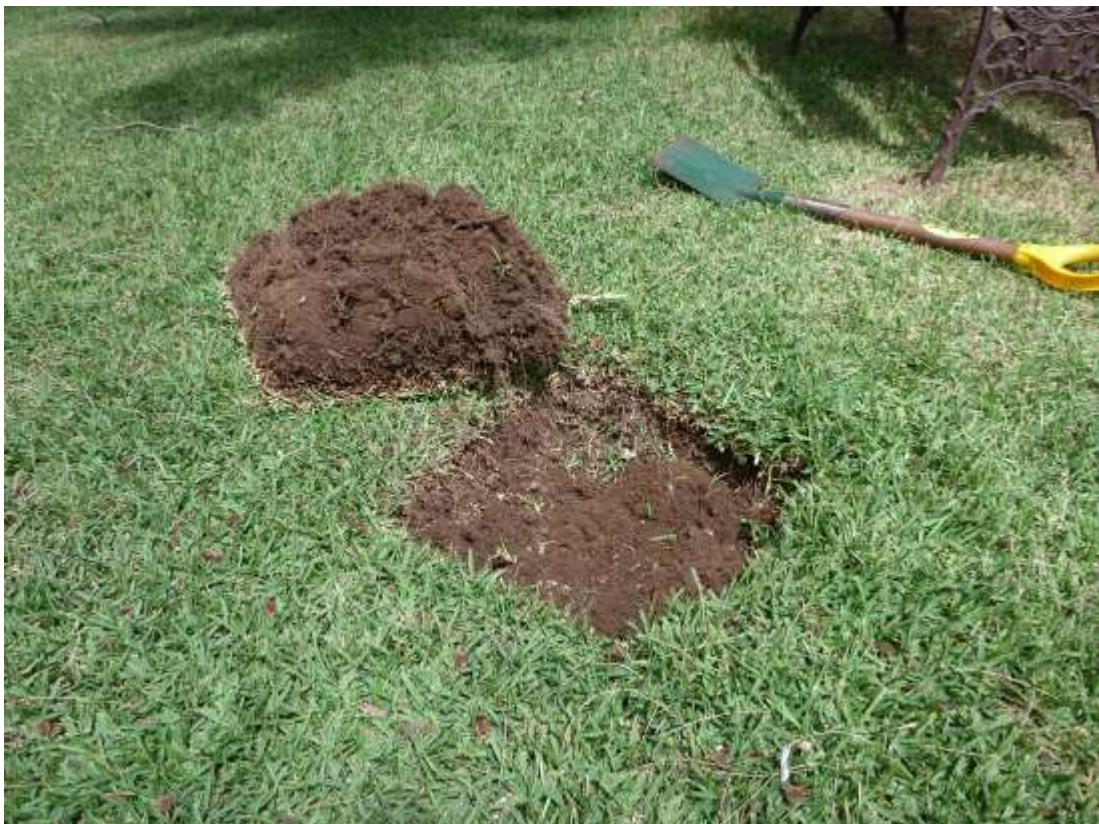
Photograph 1 – Shallow Test Pit behind the existing sandstone wall
