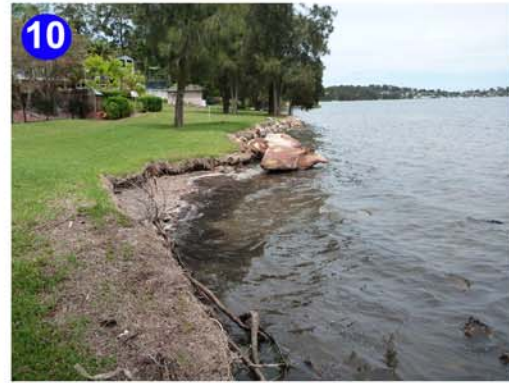
Scalloped area with 0.5m scarp. Rising main thought to lie underneath scalloped area
