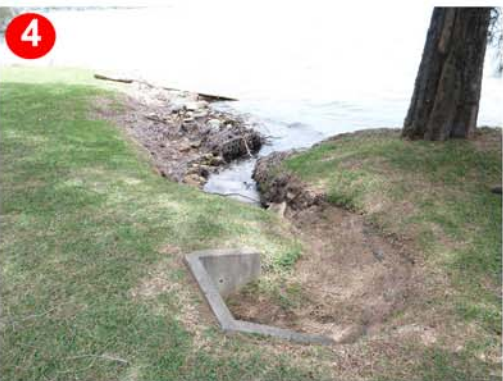
4 Pipe terminated behind seawall and dilapidated gabion
