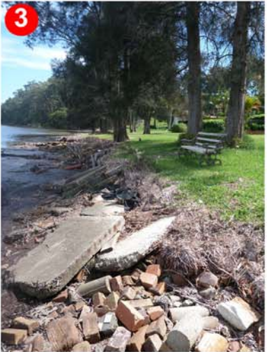
3 Brick and concrete rubble along foreshore
