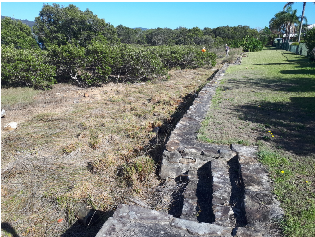
Photo 9: Same area as Photo 8 after the Juncus was treated.
